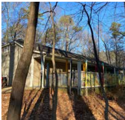
Studio School Building
